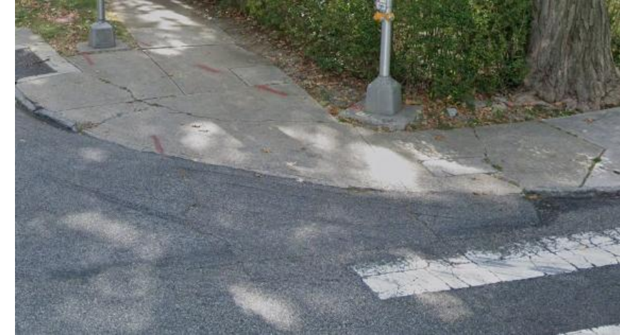
Top Left: non-APS push button with missing sign on NE corner of Montgomery Avenue & Roberts Road.
