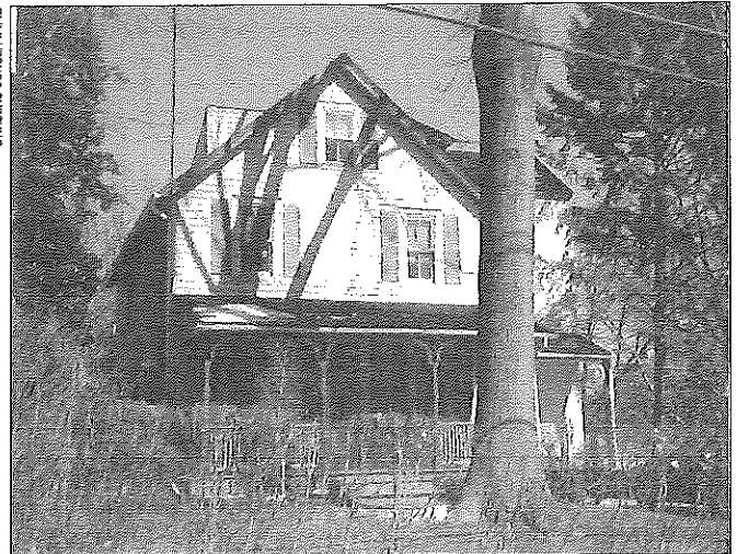
Following severe fire damage, a house returned to its previous appearance after repair and replacement.
