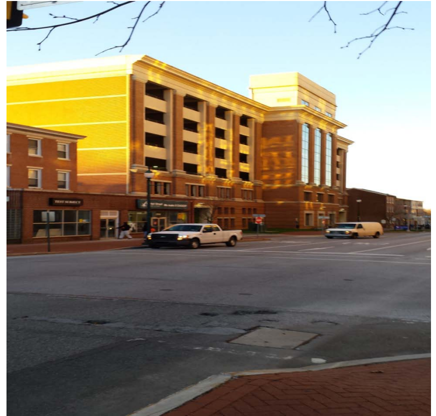
COUNTY JUSTICE CENTER GARAGE
